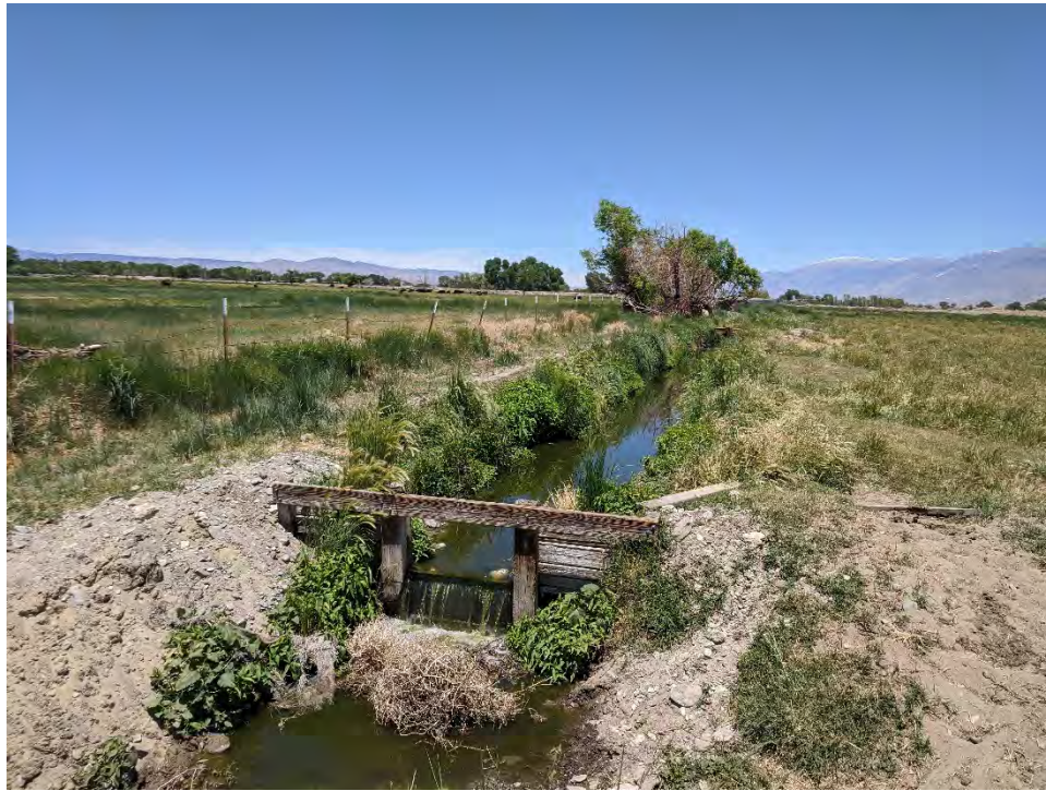
Photo 9: Representative view of a drainage ditch containing water, running north to south from the wastewater treatment plant through Phase 1 of the Study Area. Date of photo: May 27, 2021.
